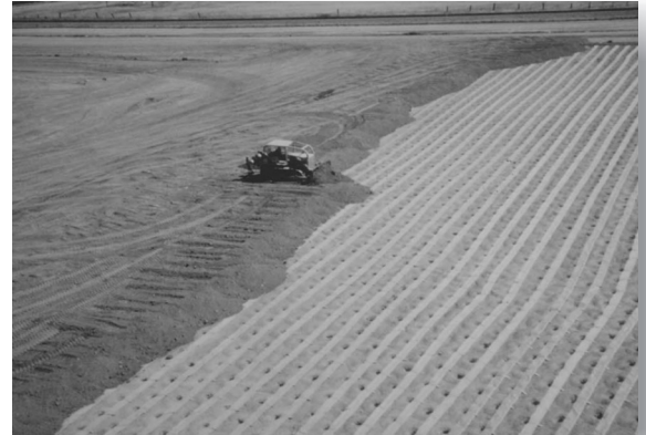
Wick drains and strip drains being covered by surcharge layer.
