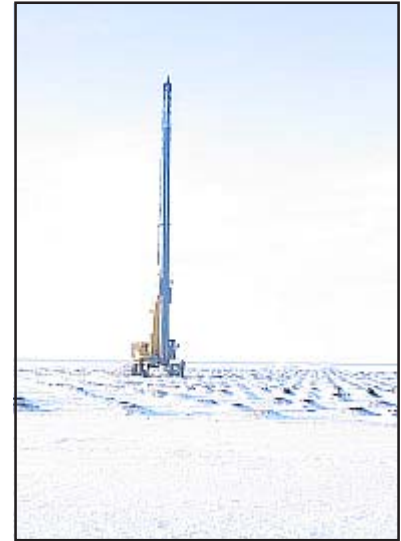
Figure 3: Installing wick drains on the wick drain pad.
