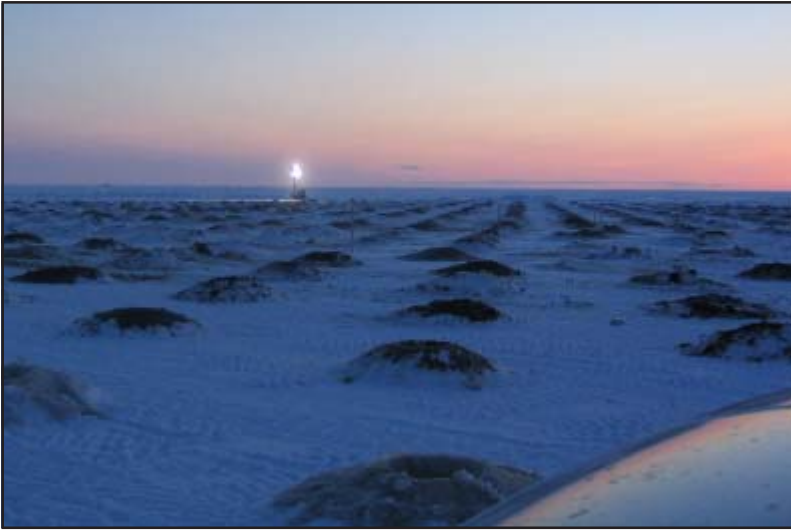
Figure 2: Preaugered holes drilled through ice prior to wick drain installation.
