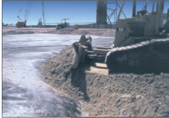
Construction of "Finger Fills." Left: Using the bulldozer. Below: Using broadcasting.
