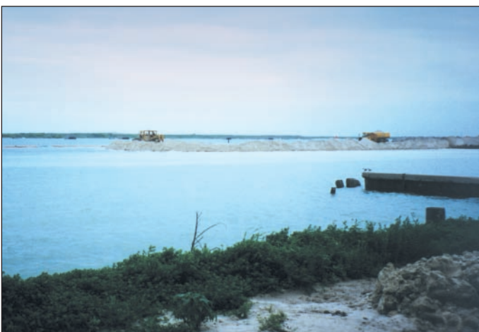
Construction of closure dike.
