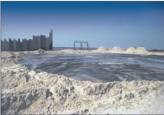
Geotextile deployed and anchored.
